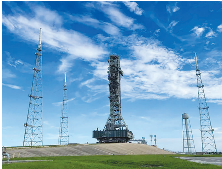
Mobile Launcher 1 crawls toward Launch Pad 39B
